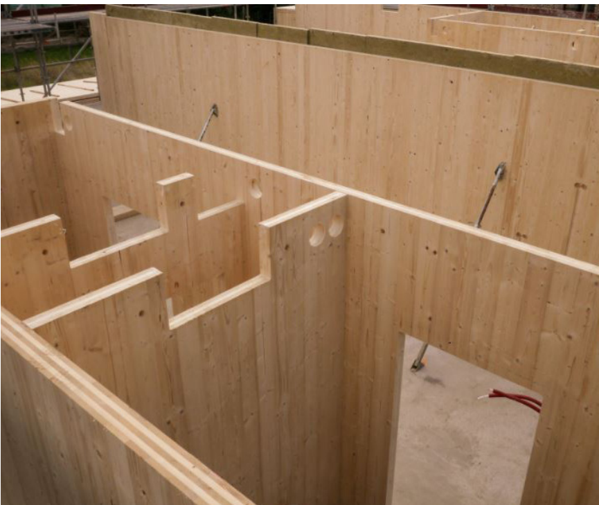
cross laminated timber (CLT) binnenwanden
