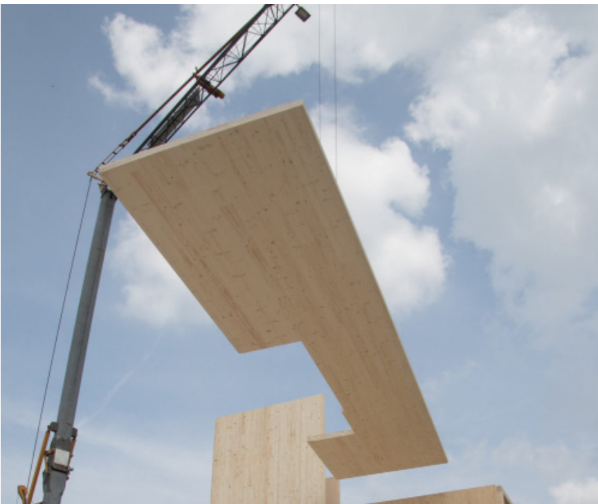
cross laminated timber (CLT) vloerdelen
